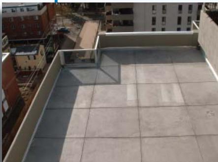
Concrete placed over Drain Matt System
